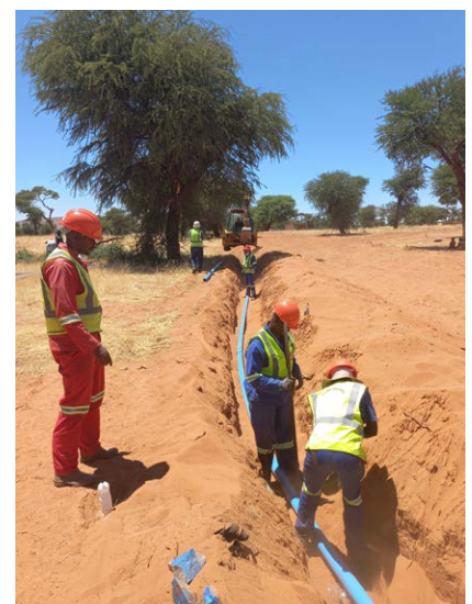
Construction of the water reticulation network in the Rehoboth project area.
