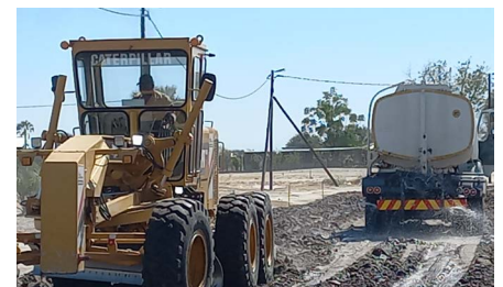
New road being constructed to the Oniipa project area
