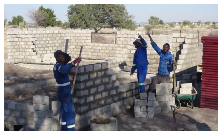
First houses being built in Onawa Extension 9
