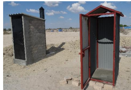
Metal toilet hut (right) built locally, to be connected to a septic tank that has been constructed in the back of the hut. These two sanitation solutions were built in the Okahao project area.
