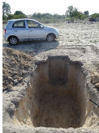
Left: pit excavation for the ‘Okakedi’ pit latrine in Oshakati.
