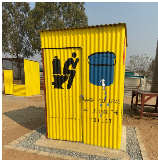
Newly constructed sanitation centre with business stall in Max Mutongolome (Windhoek)
