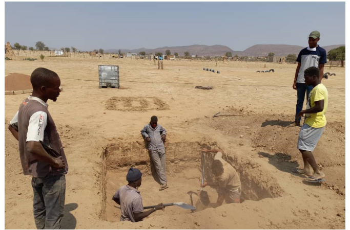
Construction of pit for a new sanitation centre in Opuwo
