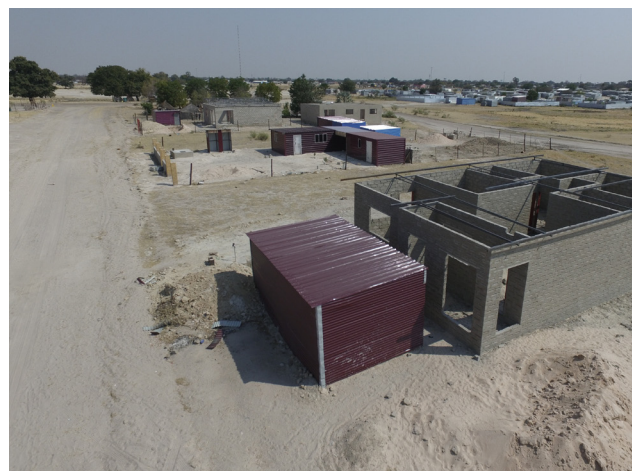
Homes in different stages of construction in the Oshakati layout
