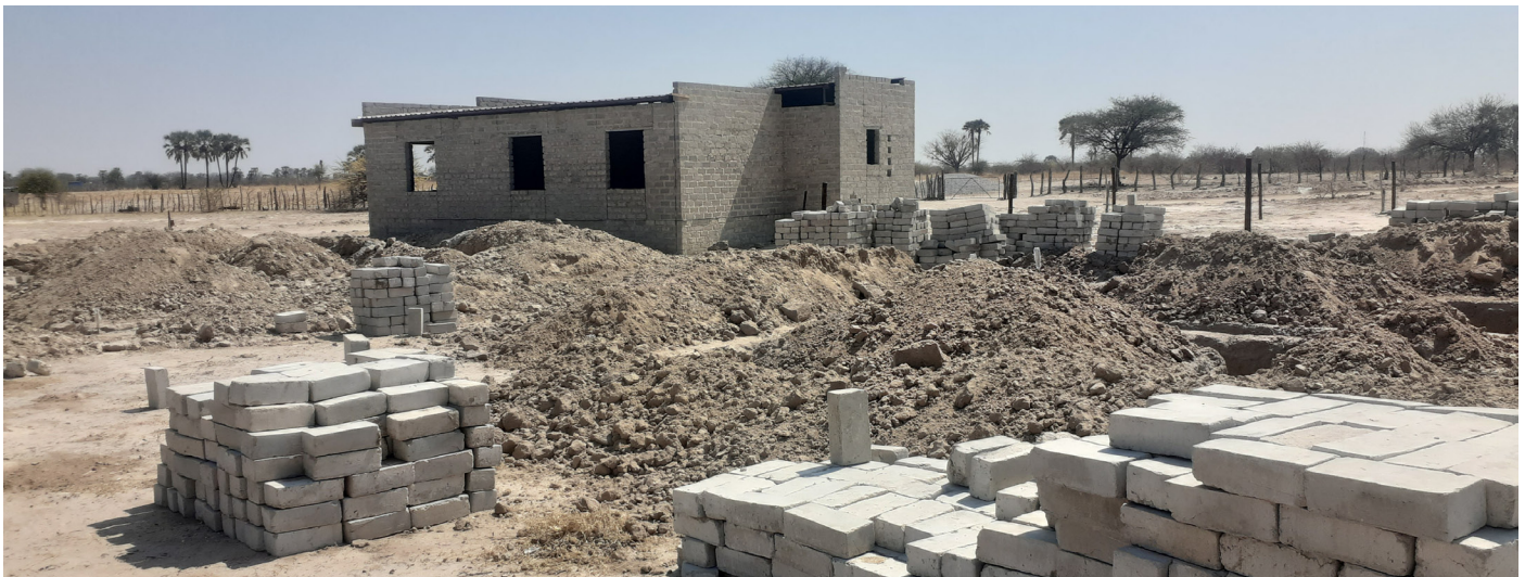
Housing construction in Okahao
