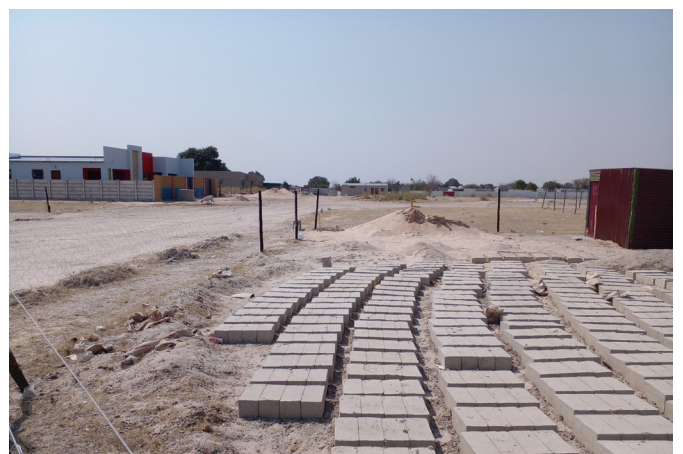
Brick production in Oshakati, with the owner preparing the construction of the first phase of the house
