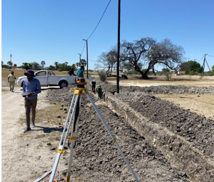
Preparing excavated trenches for water pipes.
