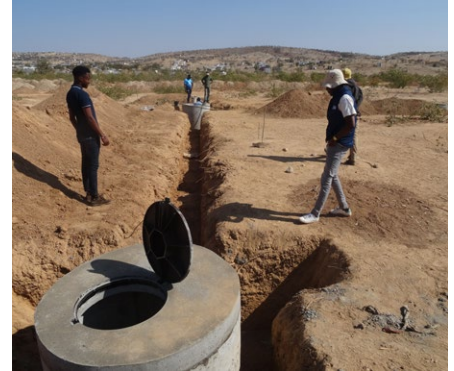
Site inspection by DWN staff in Opuwo
