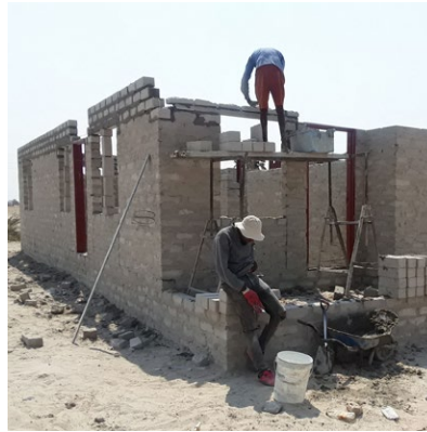
House being built in Okahao
