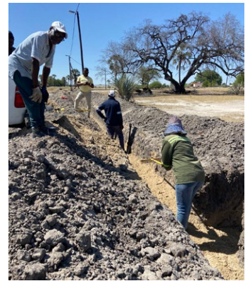
Trench preparation for water pipes in Oniipa
