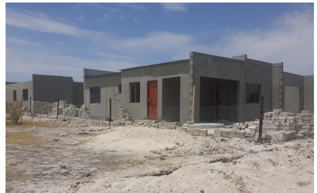
New houses are being built in the Oshakati project area
