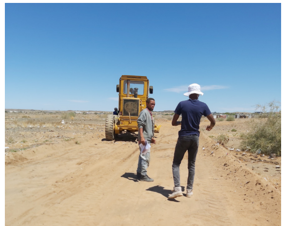
Road blading of the layout in Keetmanshoop
