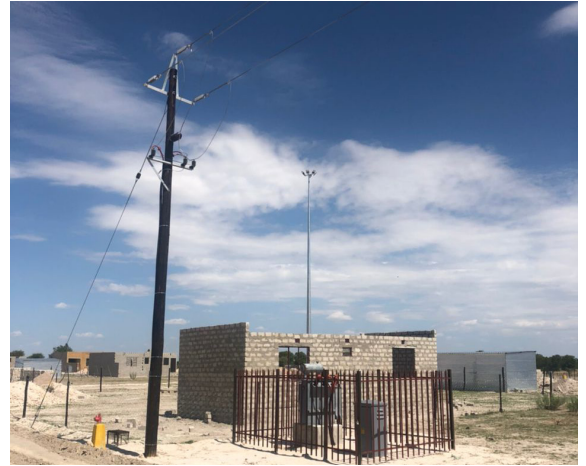
The first project area in Oshakati is now fully electrified.
