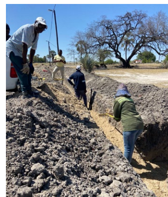
Trench preparation for water pipes in Oniipa
