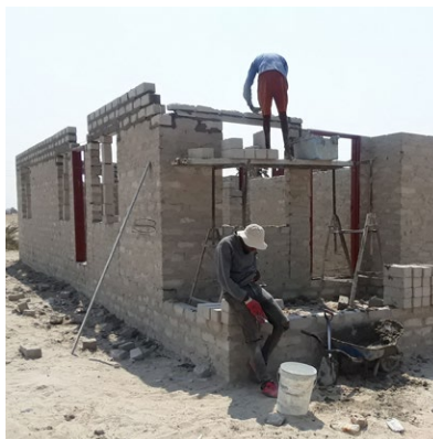
House being built in Okahao
