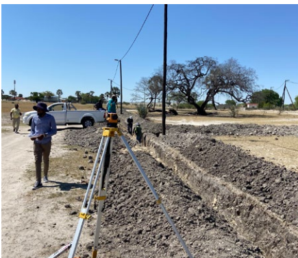
Preparing excavated trenches for water pipes
