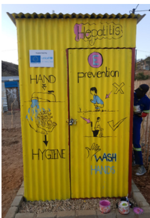
Toilet built at an ECD centre.
