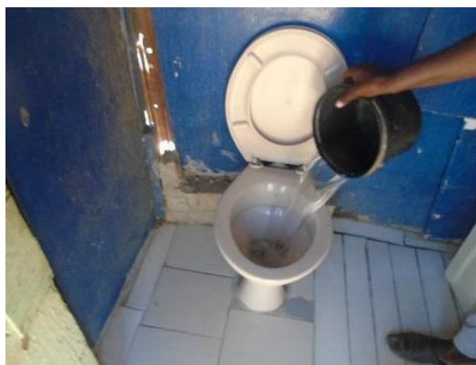
Pour flush toilet with seepage pit in Havana informal settlement, Namibia
