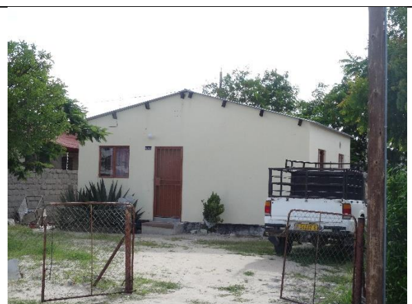
House in Uupindi informal settlement in Oshakati
