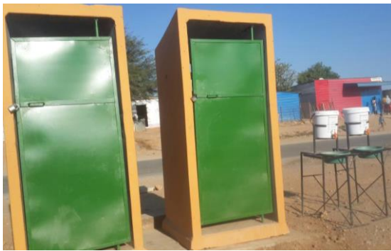
Community flush toilets in informal settlements in Windhoek
