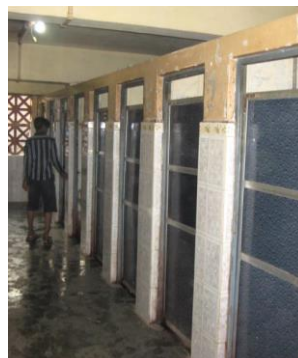
Toilet cabins (India)
