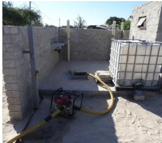
Conservancy tank in Oshakati informal settlement, being emptied by a 'honey sucker'
