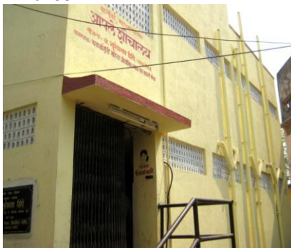
Community toilet block structure (India)
