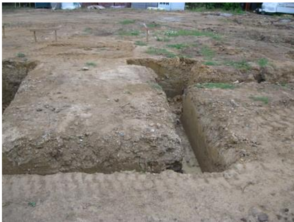
Figure 5: Foundation Trenches (setting out and foundations dug. (weebly.com))
